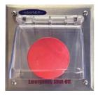
Remote Emergency Shutoff Button Automatically turns utilities off.
